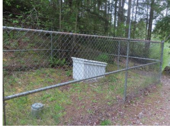
Typical Chain Link Fence Surrounding Well
