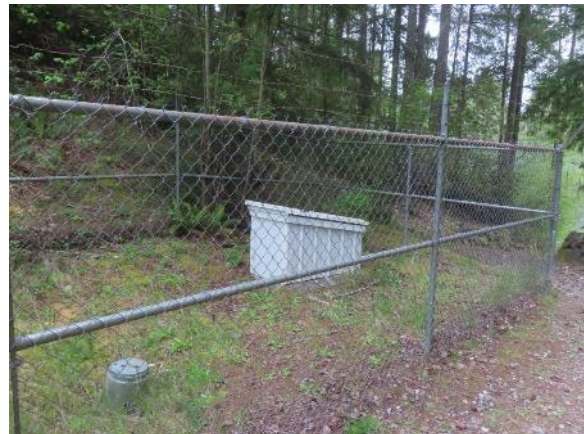
Typical Chain Link Fence Surrounding Well
