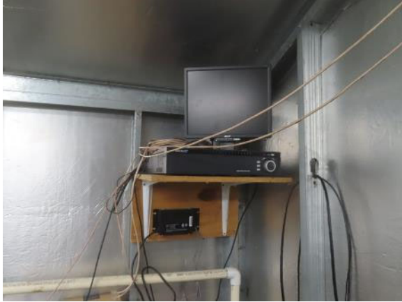
Surveillance System Recording Equipment and Monitor
