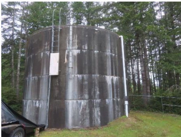
Concrete Water Storage Tank
