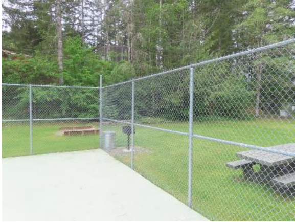
Chain Link Fence Surrounding Sport Court
